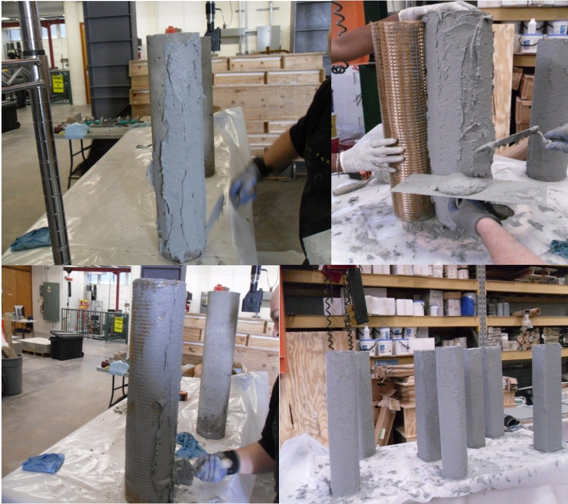
Fig. 4-2: Demonstration of installation procedure of PBO-FRCM strengthening
