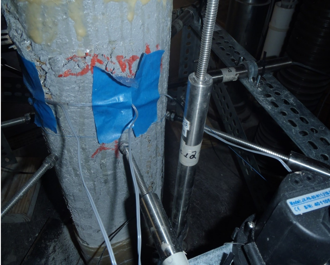
Fig. B-12: Failed PBO-FRCM wrapped circular column
