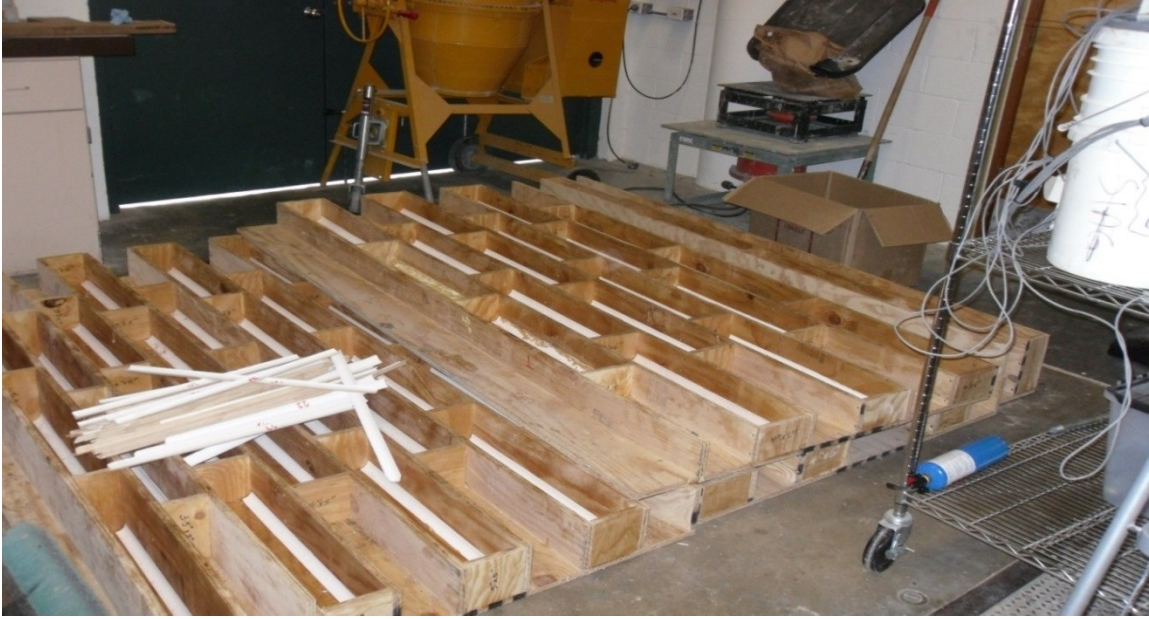
Fig. B-2: Formwork
