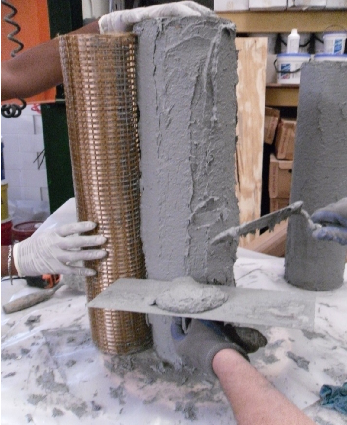
Fig. B-7: Application of the PBO fiber
